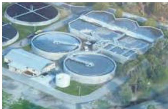
Figure 10.7 An aerial view of a sewage plant
