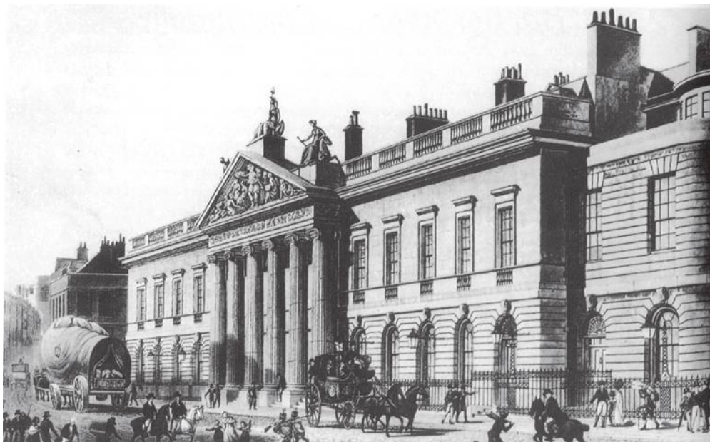
Fig. 17 – East India Company House, London.
