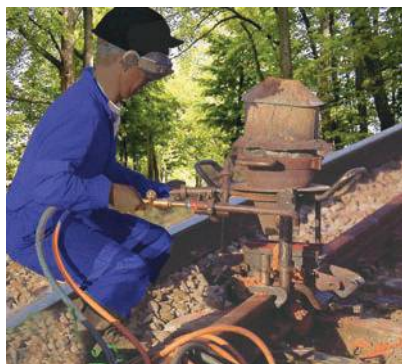
Figure 3.11 Thermit process for joining railway tracks
