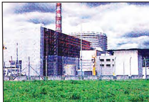
Fig. 3.16 : Nuclear power station , Kalpakkam
