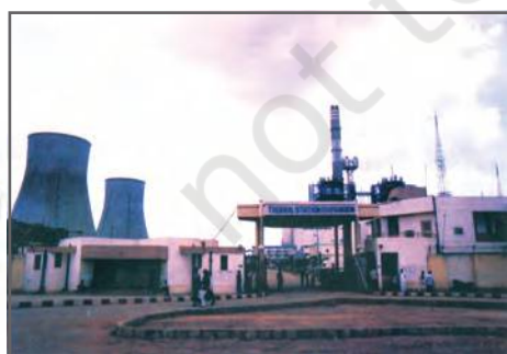
Fig 3.10: A view of a Thermal Power Station
