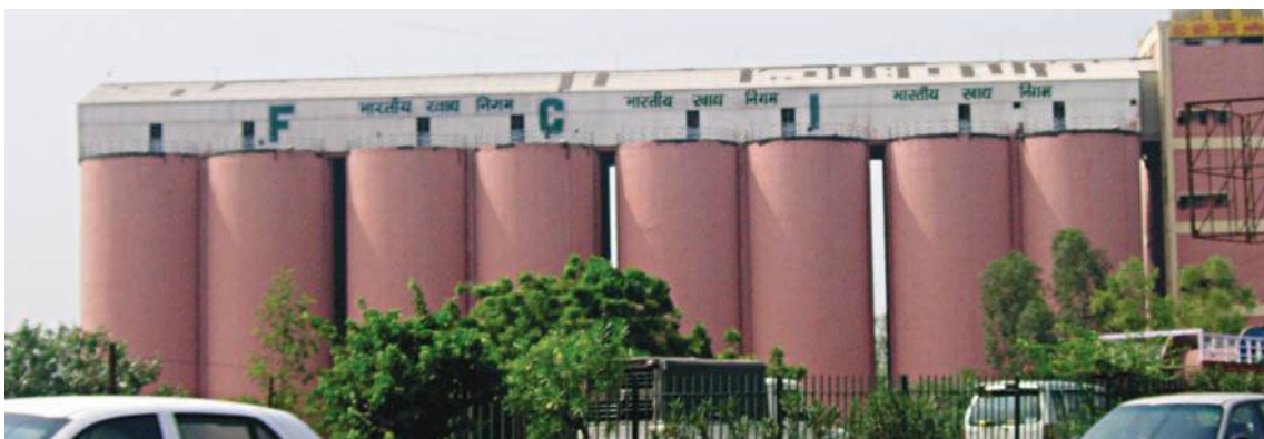
Fig. 1.10 (a) : Silos for storage of grains
