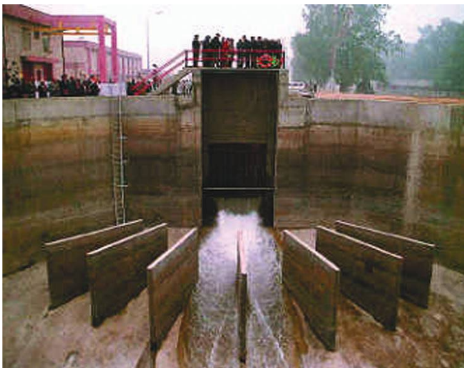
Fig. 18.10 : Water treatment plant
