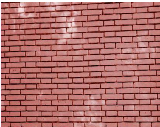
(a) Brick wall
