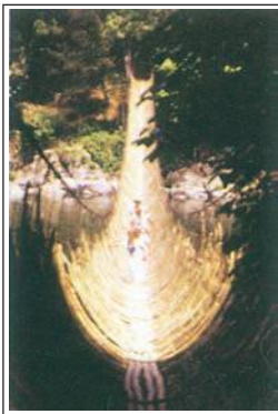
Figure 6.7 : Rope Bridge (Arunachal Pradesh)
